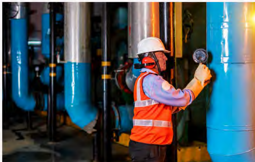
➤ Sewage treatment plant
