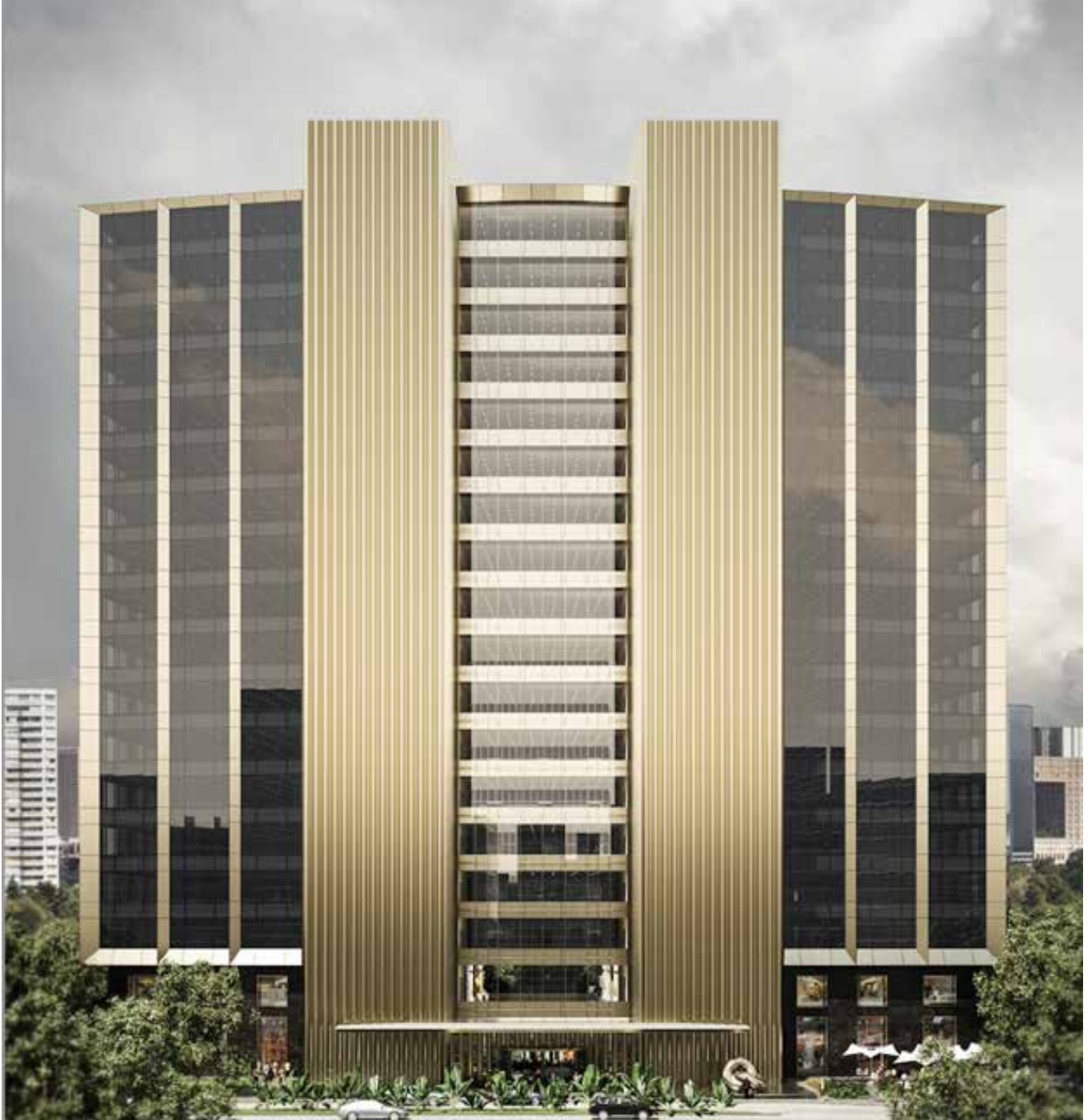
↖ The Tower 11 executive entrance facade: An amalgamation of brass and black mirror details to exuberate regality and monumentality
